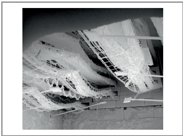
Fig. 4. Interior of a test chamber 25 min after commencing the DIN 4102-12 test. Temperature equals approximately 820°C. The sagging of cable trays is already considerable. The photograph was taken at the FIRES test lab in Batizovce, Slovakia, in 2019. Photo courtesy of Krzysztof Borzycki.
